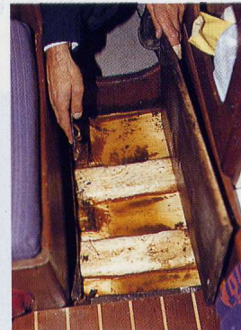
Check for corrosion of the steel keel fastenings. Hairline cracks in the reinforcement indicate stress
